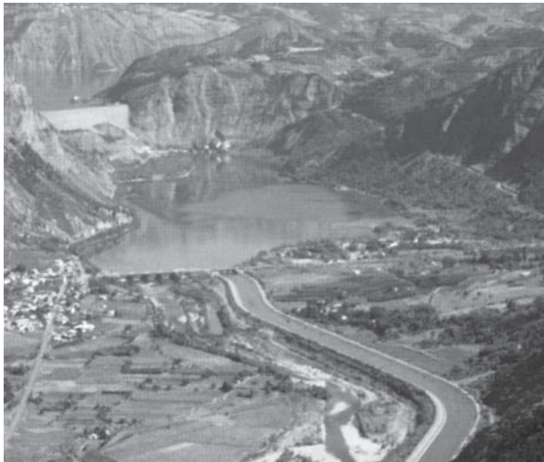
Figure 1: Example of a hydroelectric scheme (Photography: all rights reserved). Background: a water retaining scheme (Serre Ponçon dam); foreground: the upper part of a water diversion scheme (Espinasses dam and Durance channel).
